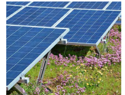
Elevated PV panels above living roofs
