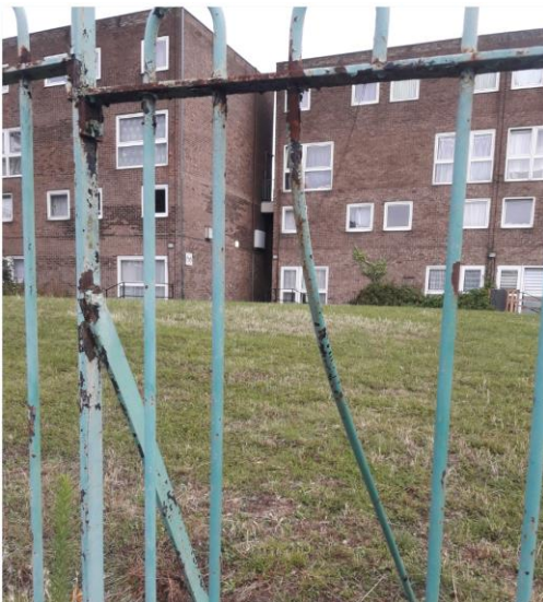
4.1 and 4.2 broken and missing railings on fences behind Whitehall Street flats
