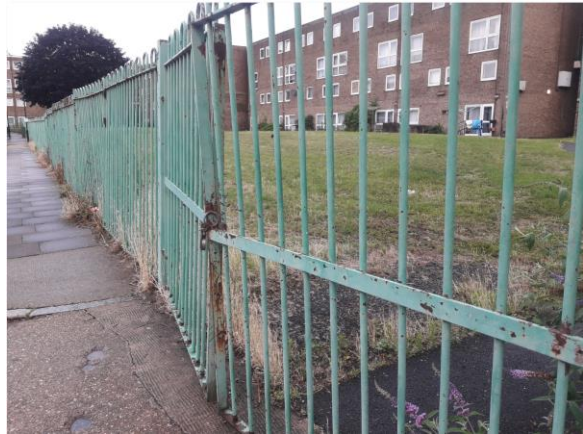
4.3 and 4.4 rusting fencing and damaged gate in railings behind Whitehall Street flats
