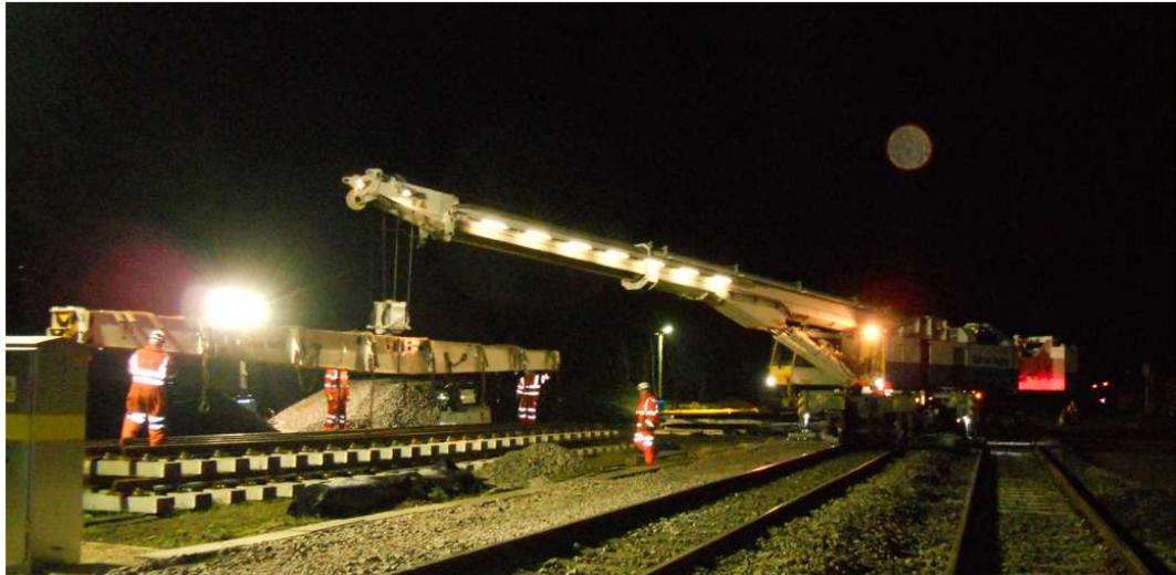
Figure 48: Kirow 1200 lifting S&C Panels
