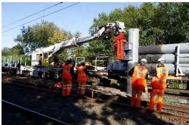
Figure 51: Piling train arrangement
