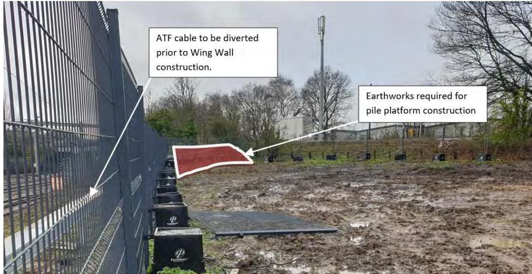
Figure 89: Piling platform location
