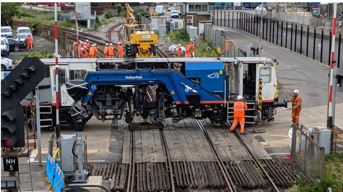
The Beaver tamper is rotated on a pivot at the middle of the machine as seen in the photograph. The workers can then push it round facing the right direction.
