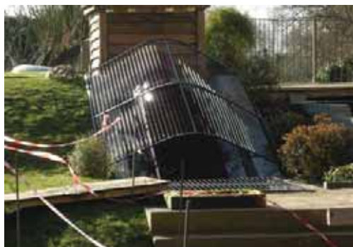
Fig 7.8: Archimedes screw, hydro generation, East Hanney
