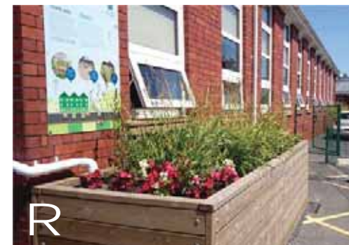
Fig 3.14: Dowpipes diverted so that rainwater drainage can be used to irrigate planters
