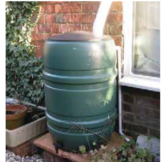
Fig 7.10: Water butts are simple solutions to recycle rainwater
