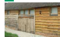
198 Replacement weather board
