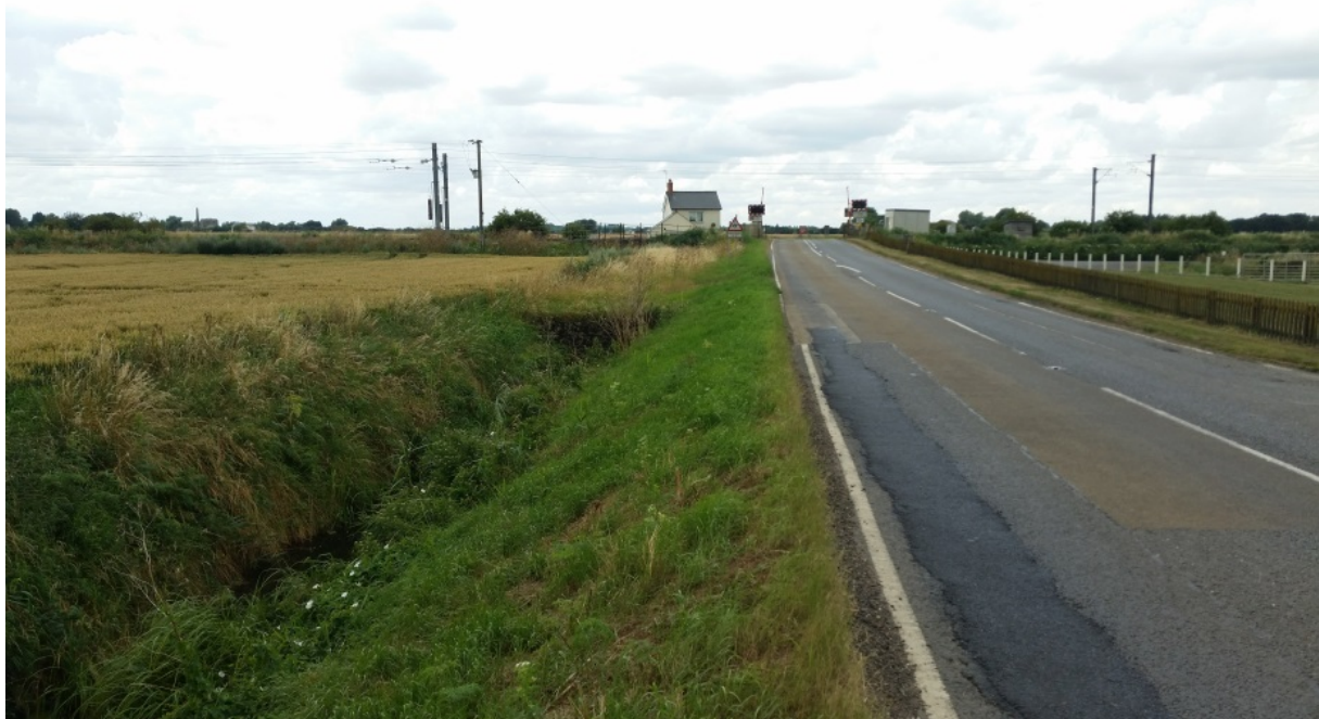
Figure 2.1: Narrow carriageway and verge with steep embankment.
