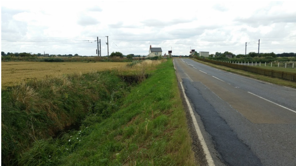
Figure 2.1: Narrow carriageway and verge with steep embankment.
