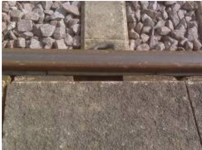
Figure 11 – Bomac 113A wedges installation
