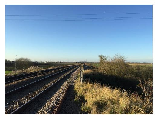
19.13 As can been seen from the table above (19.8), C16 Prickwillow 1 level crossing does not have sufficient sighting to meet industry standards for up side looking toward up direction train approaching and down side looking toward up direction train approaching in these directions is heavily restricted by railway underbridge 1579a and is limited to 10 metres.C16 Prickwillow 1 level crossing has whistle boards installed as a mitigation measure for insufficient sighting.
