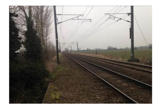
34.13 As you can see from the table above (34.8), C35 Ballast Pit level crossing does have sufficient sighting to meet industry standards in all directions. C35 Ballast Pit crossing is on a long straight section of the railway as shown in the photographs above. This means the sighting for a user to see an approaching train is very good
