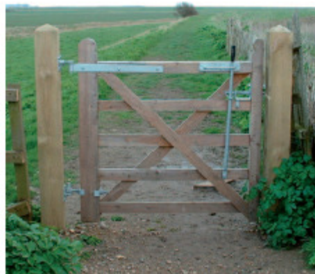
Figure 17: G1 Wooden Footpath Gate Example
