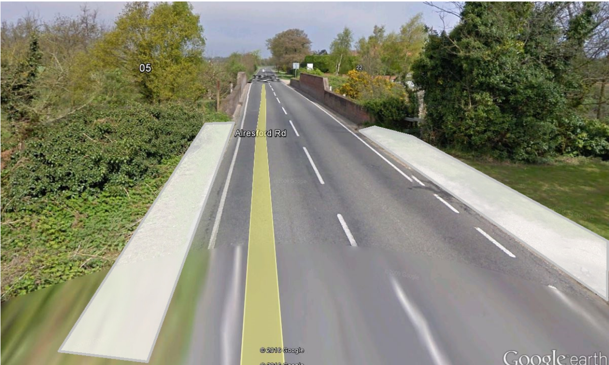
Figure 55: Sketch of verge hardening on bridge approaches
