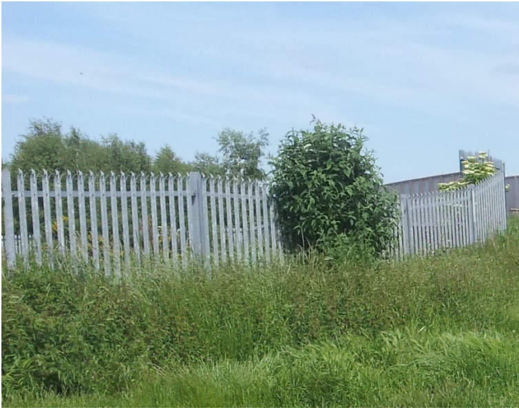
Figure 15: Illustrative example of Steel Palisade Security fence
