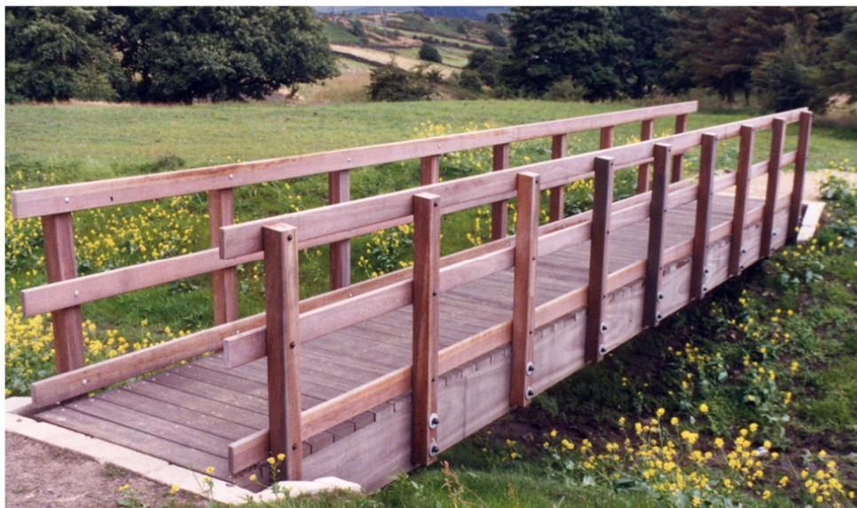
Figure 41: Illustrative example of footbridge (with Timber parapets) Type E-B3
