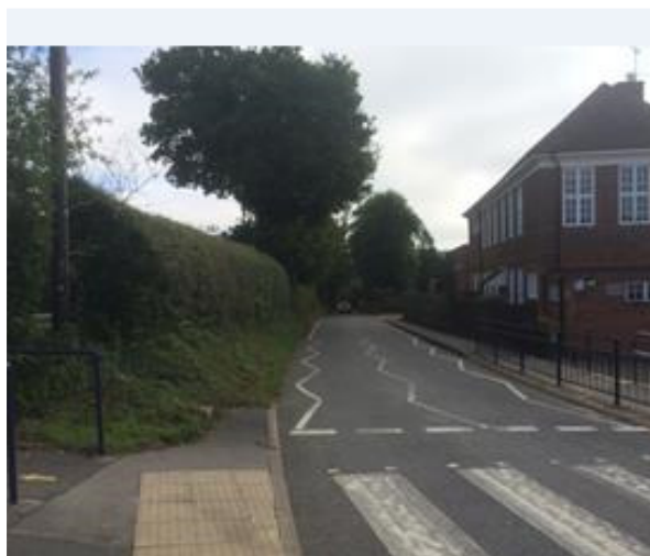
Figure 31: Tactile crossing example
