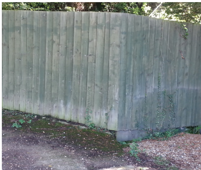
Figure 13: Illustrative example of Close Boarded Wooden Fence
