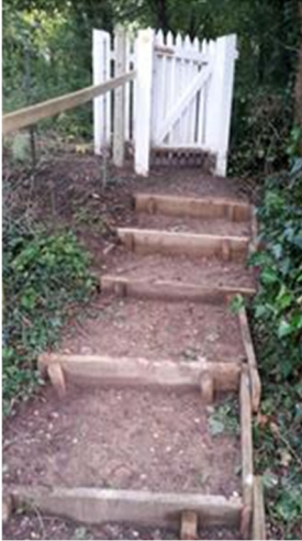
Figure 45: Illustrative example of timber board steps
