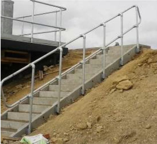
Figure 49: Illustrative example of concrete modular access steps
