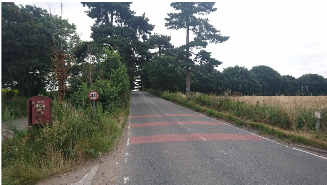
Figure 2.18: Lack of verge or footway on Ockendon Road.
