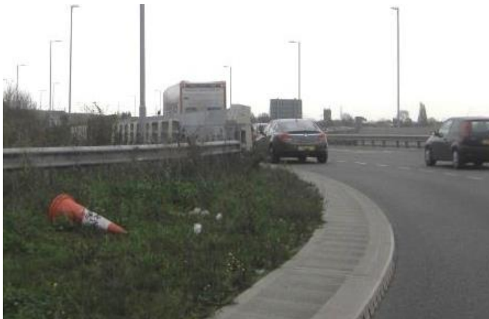
Figure 2.7: Proposed footway behind safety barrier.
