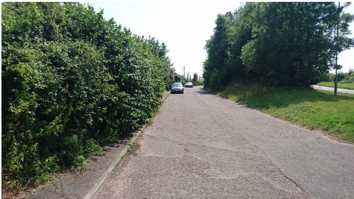
Figure 2.5: Overgrown footway along back of layby.
