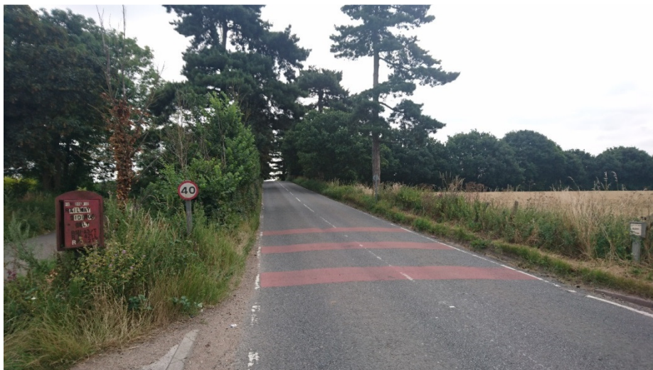
Figure 2.17: Lack of verge or footway on Ockendon Road.
