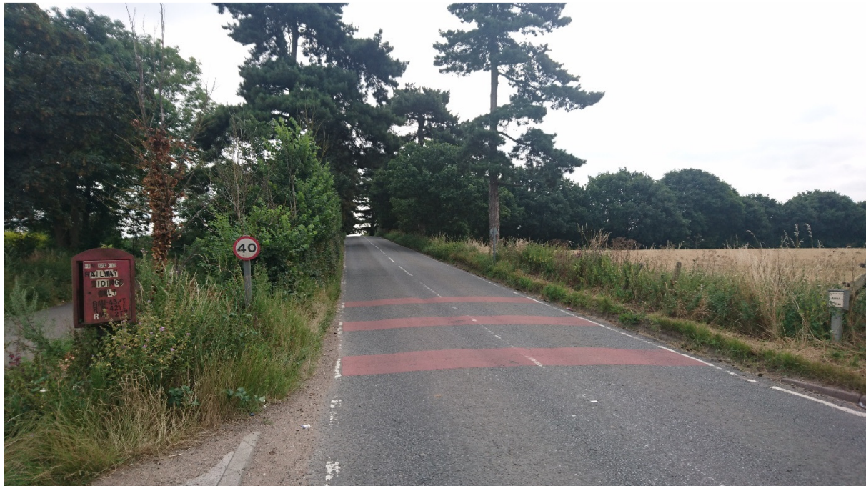
Figure 2.2: Lack of verge or footway on Ockendon Road.
