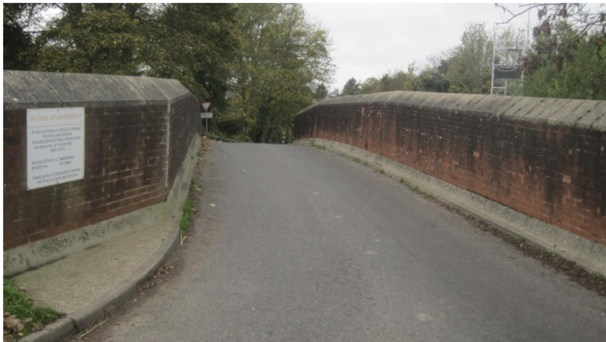
Figure 2.2: Restricted width on Debden Road over railway line.
