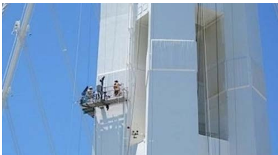
Figure 10: Use of inspection gondola on inclined tower faces of San Francisco-Oakland Bay Bridge
