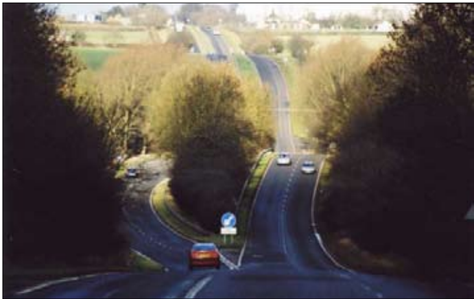
Figure 8.7 Sensitive vertical alignment that respects the topography of the local historic landscape. Left A5. Right A46 north of Leicester © Scott Wilson Limited.
