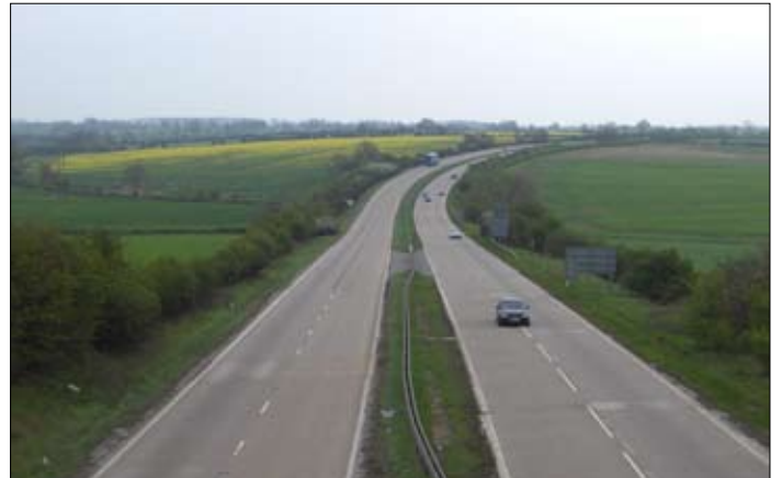
Figure 8.7 Sensitive vertical alignment that respects the topography of the local historic landscape. Left A5. Right A46 north of Leicester © Scott Wilson Limited.
