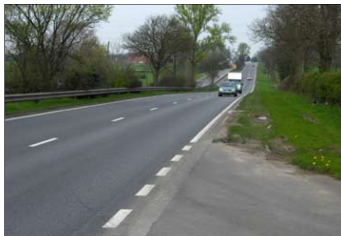
Figure 8.2 Benefit of asymmetrical widening and retention of existing boundary as central reservation in dual carriageway design – Left A417. A retained mature central reservation may help to integrate roads into their historic landscape surroundings © Halcrow Group Limited – Right - A46 Leicester © Scott Wilson Limited.
