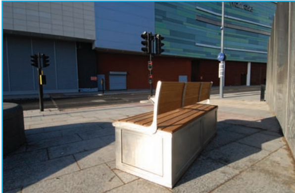
Bench containing traffic signal controller
