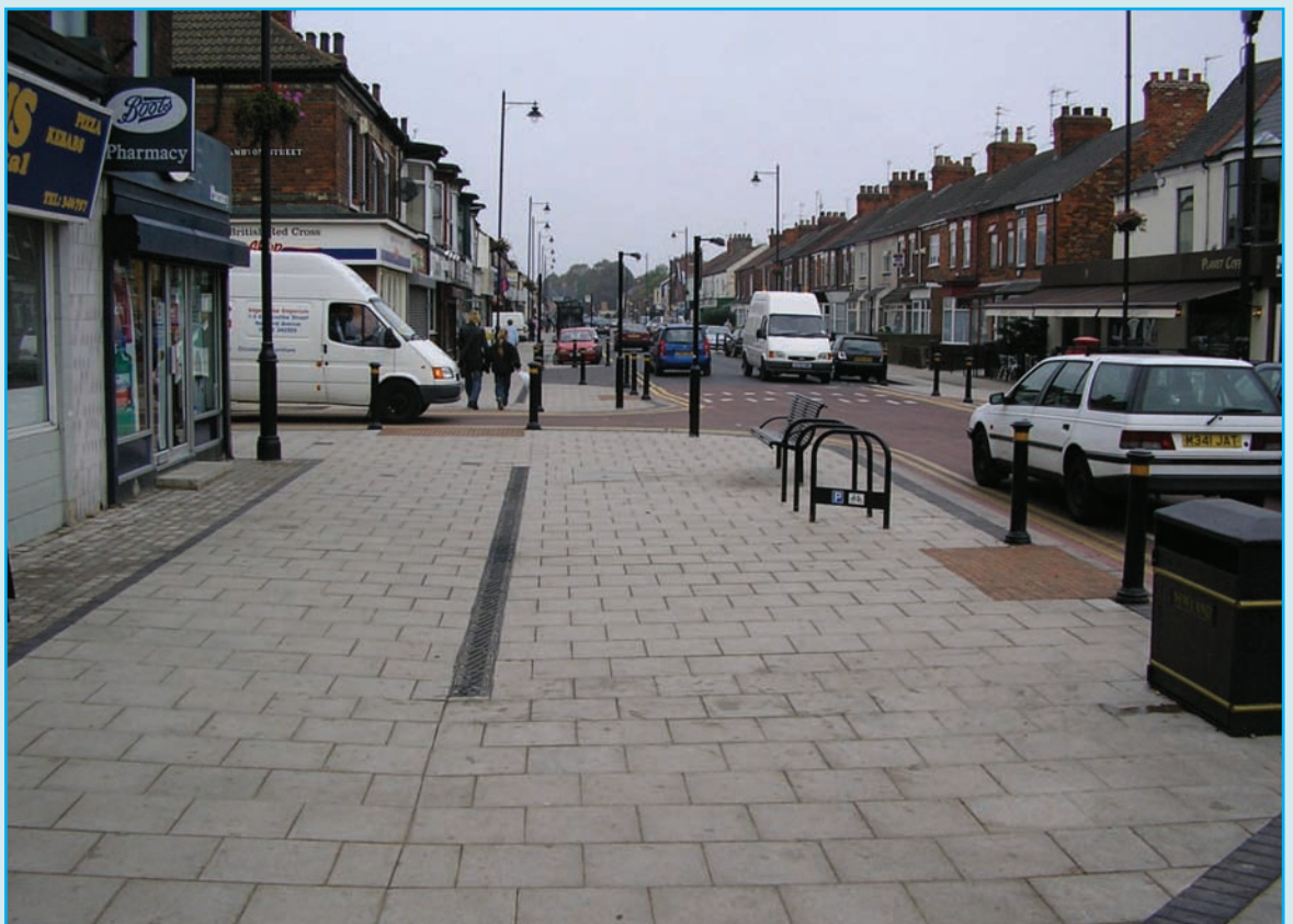
Footways widened significantly by narrowing carriageway
