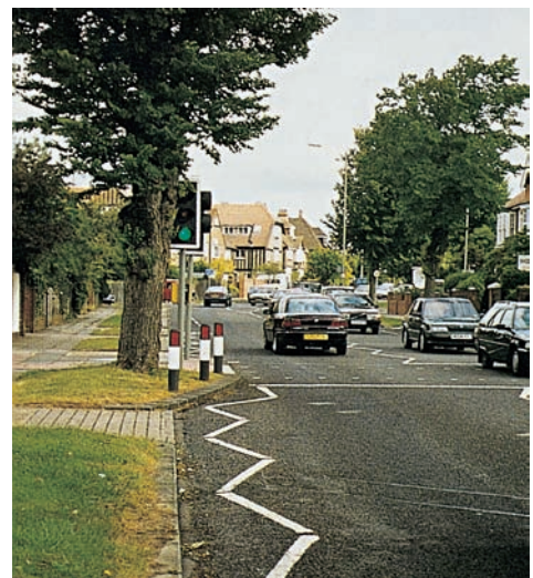
Built out kerb to improve the sight lines.
