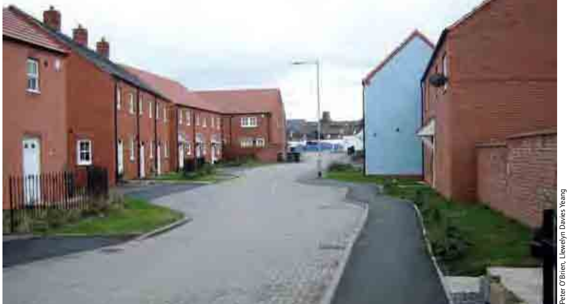
Figure 7.14 This street avoids the use of vertical traffic-calming features, but the irregular alignment is unsightly and unlikely to have much speed-reducing effect, because of the width of the carriageway. It also results in irregular grassed areas that create a maintenance burden while contributing little to street quality.
