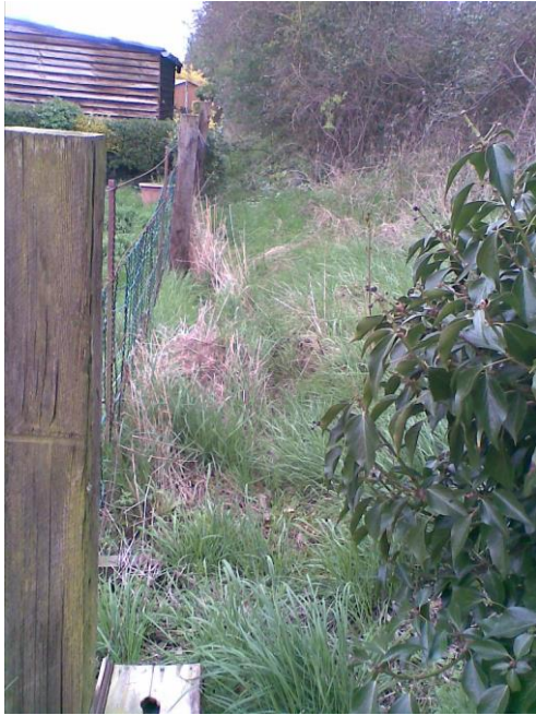
The outfall from the chamber is to the drain at the toe of the embankment. View along the inside line of the Network Rail fence showing ditch silted up and overgrown with grass.
