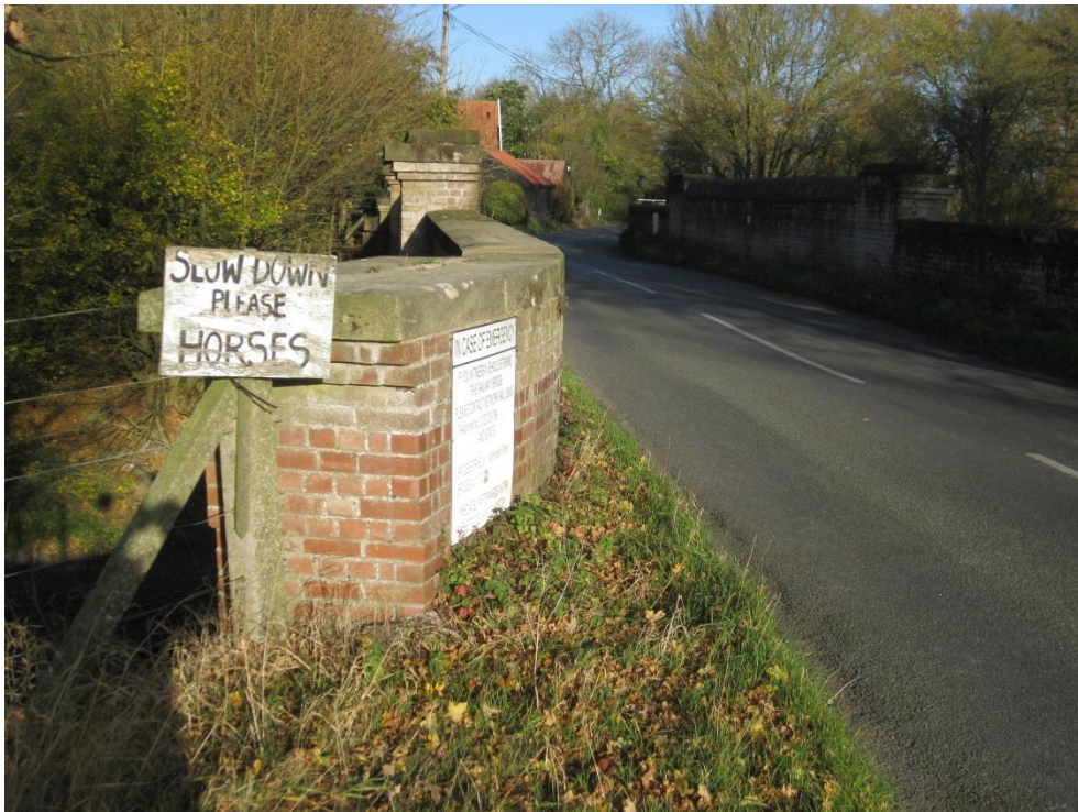
Photo C: narrow road bridge, no footway and no refuge—
