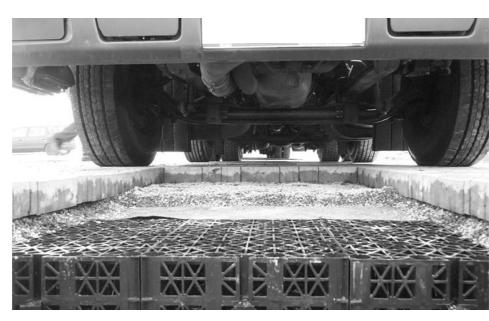
Figure 9.13.1 Plastic modular storage tank below a trial car park at Coventry University. View taken during deconstruction at the end of a one-year trial (SEL Environmental Limited)
