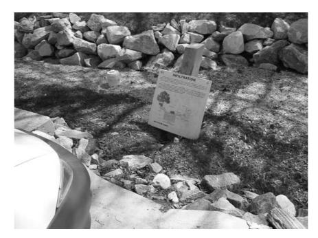
Figure 9.8.1 Infiltration trench
