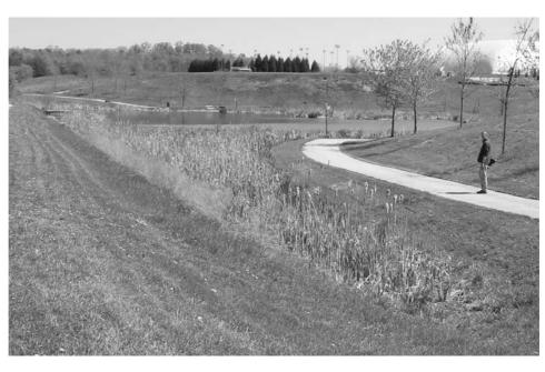
Figure 9.7.8 Swale integrated into landscape and retention pond
