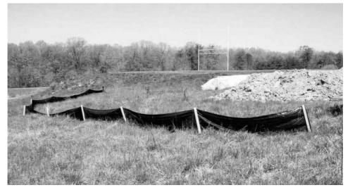
Figure 6.1 Geotextile silt fence to remove silt in runoff
