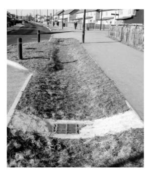
Figure 9.7.1 Swale in a housing development, Scotland
