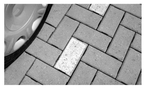
Figure 9.2.1 Pervious pavement
