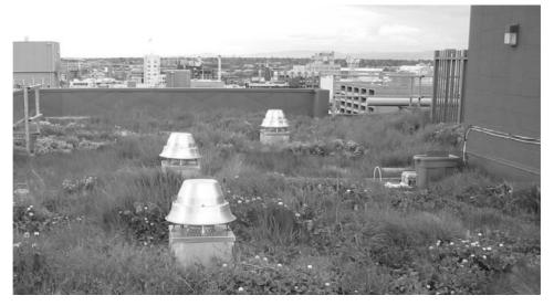
Figure 9.3.1 Extensive green roof
