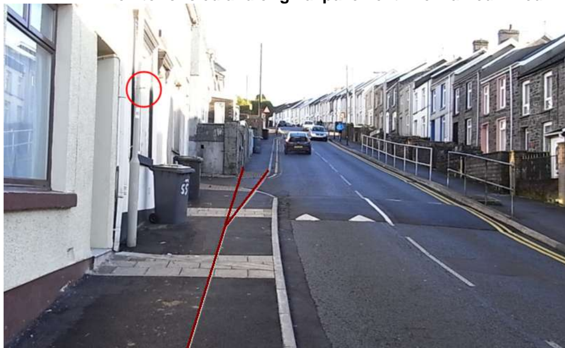
Figure 10 Traffic calming measures including pavement widening on Twynirodyn Road, Merthyr Tydfil, to modify the flow of traffic and improve driver behaviour, with air quality monitor circled and original pavement line marked in red
