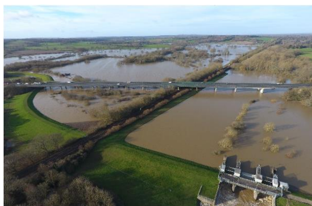
Photo 1: Leigh FSA during operation in February 2020 – Main Embankment and Control Structure visible in the foreground
