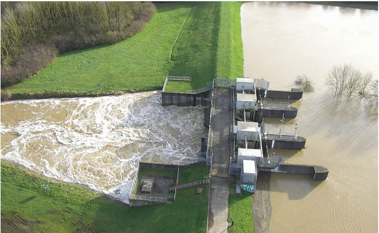
Figure 1. The water control structure and embankment at the Leigh Flood Storage Area during operation in February 2020
