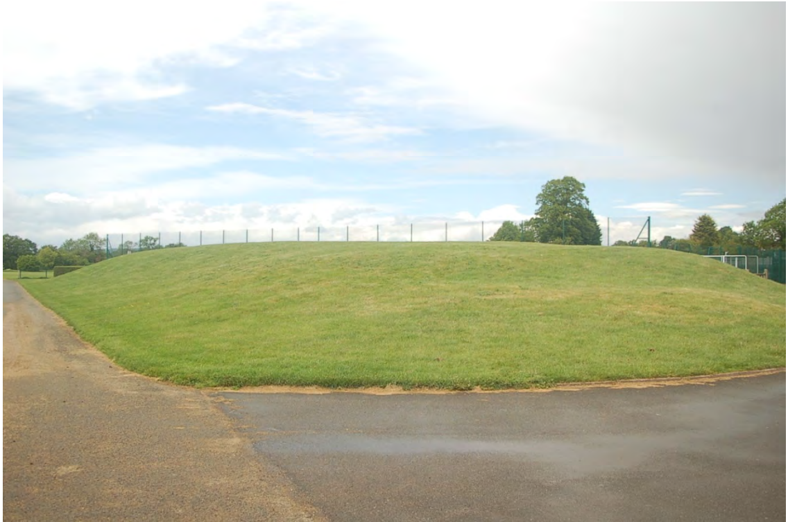
Photograph 8: Spoil heap in the south eastern part of the Site; likely up-cast derived during construction and levelling of the sports pitches
