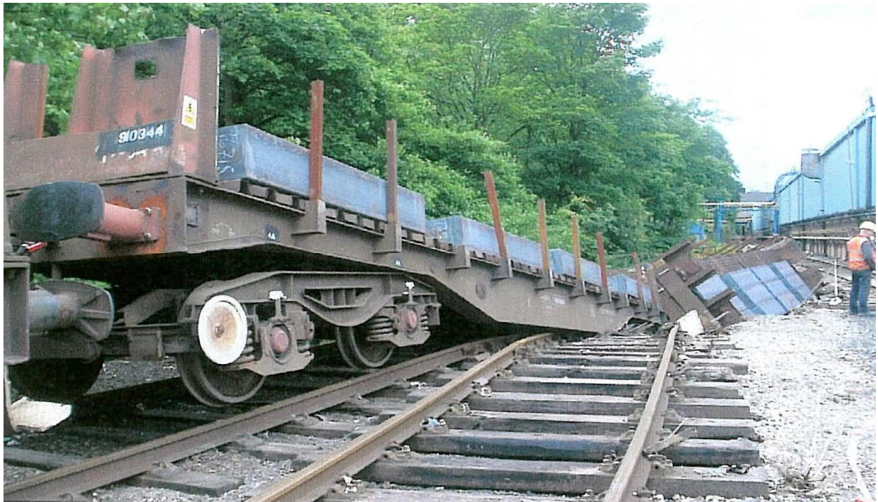
Photo 6.2: Erosion of track and ballast – Stocksbridge Steelworks following the 2007 floods
