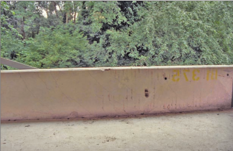
Figure 5.17 A monolithic concrete upstand restraint (after impact)
