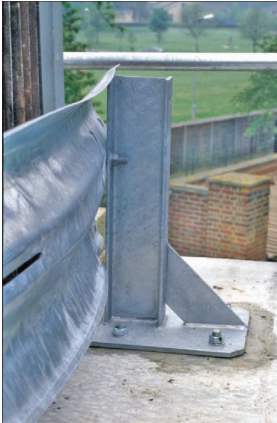
Figure 5.16 A restraint post cantilevered from the car deck (after impact on rail)
