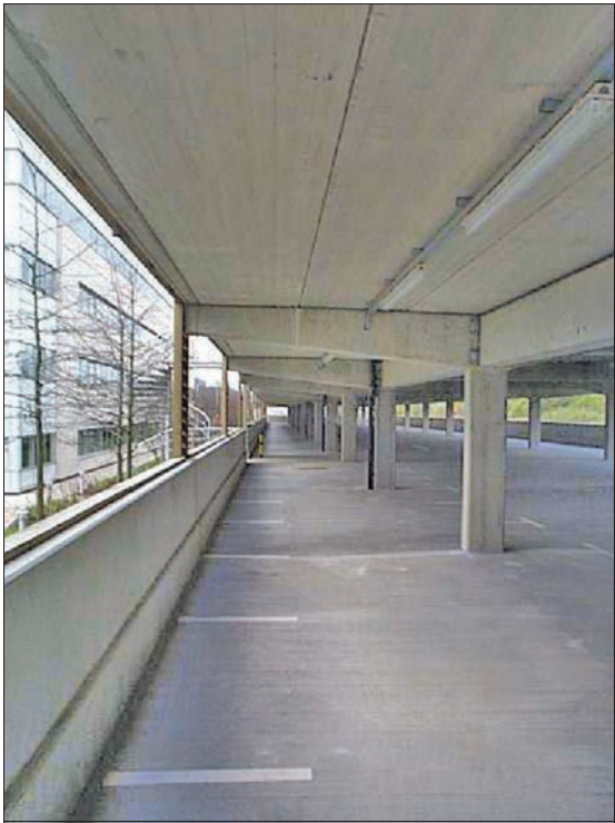
Figure 5.12 Cantilever frame arrangement
