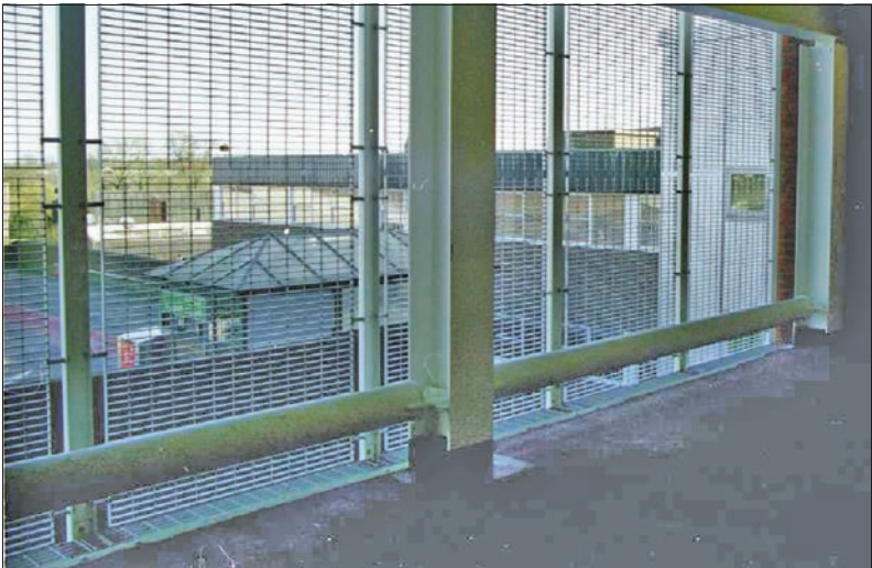
Figure 5.15 Circular hollow section vehicle restraints spanning horizontally between columns
