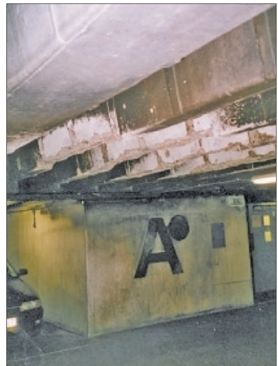
Figure 7.1 Beam damage from a car fire
