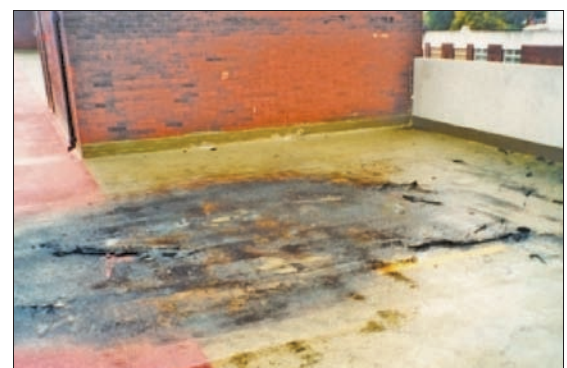
Figure 7.2 Slab damage from a car fire
