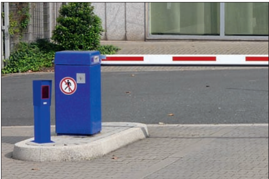
Figure 3.21 Automatic Number Plate Recognition system
