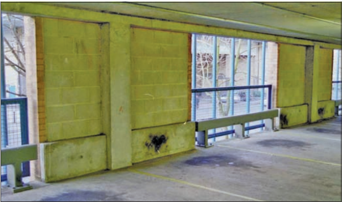
Figure 3.11 Mixed steel and concrete vehicle edge restraints, respectively fronting lightweight pedestrian restraints and masonry cladding
