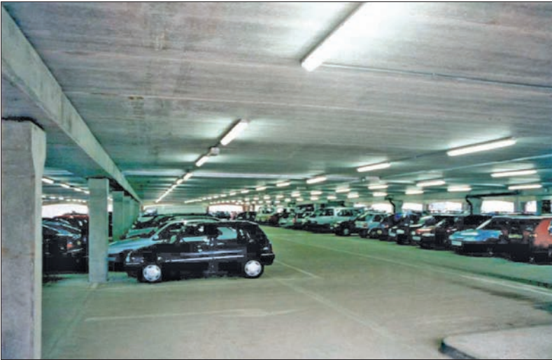
Figure 5.10 Clear span frame arrangement
