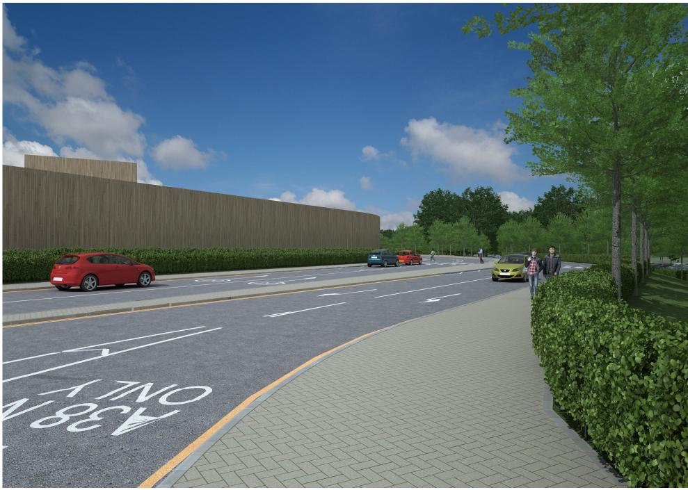
from West Lane and the controllers will be linked to ensure the operation is optimised for traffic demand. Further software and detection will be added in the form of MOVA which produce a local traffic control system which can maximise throughput and react quickly to changes in demand. The main carriageway is widened to provide two lanes in each direction over the whole of the proposed improvement, tapering back to one lane and tying onto the existing carriageway 130 metres north of West Lane.
