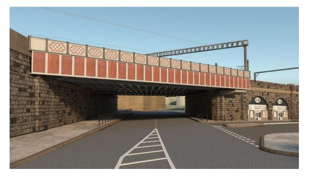
7.3.11 Span over Bradford Road. Historically the central masonry arch span was widened with metallic spans to the east and west side. The reinstatement of 4-tracking requires these spans to be brought back into use. Both metallic spans are life expired and are to be replaced with the existing arch span retained. The new spans will be of a modern form with concrete beam decks supported on new masonry clad abutment walls which will complement the existing historic features.
