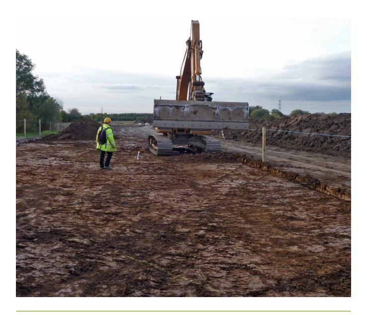
Figure 5 Construction vehicle load and rutting from wheels can cause damage to archaeological deposits.
