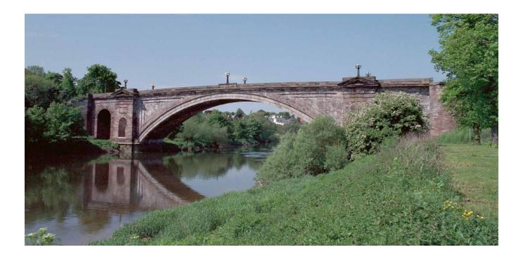
**Figure 2**Grosvenor Bridge, Grosvenor Road, Chester. When designed in 1824 by Thomas Harrison the 200-foot single span of the Grosvenor Bridge was one of the
