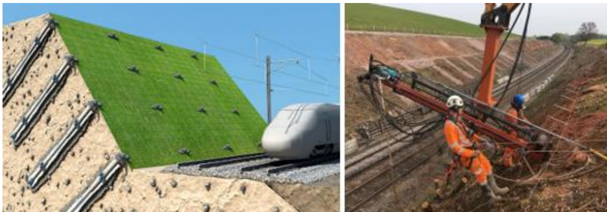
Figure 3-24: Soil nailing, concept visualisation and installation example
