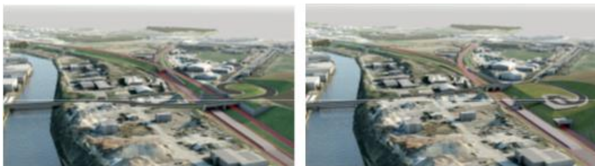
Figure 3-9: Operational Layout 1, Flyover (1A) and Dive-under (1B) Visualisations
