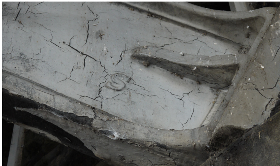
Figure 18: River Calder Bridge (MDL1/8). The detail below shows one of the letters that is believed to relate to the construction sequence
