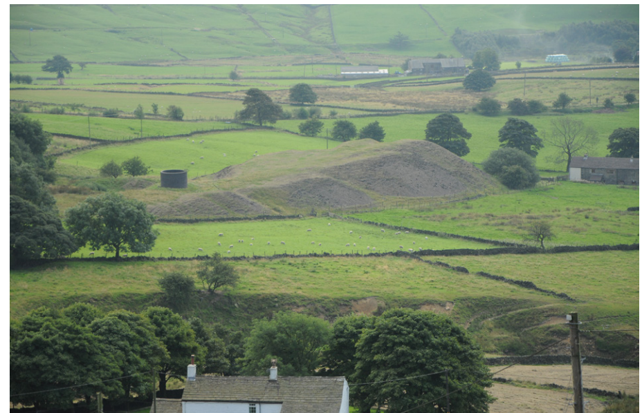
Figure 19: Ventilation tunnel (centre left) and construction spoil heap (centre), above Standedge Tunnel
