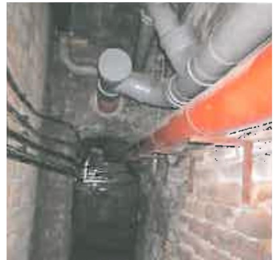
Figure 5.4.8.1c: Foul and roof water drainage within station cellar walkway
