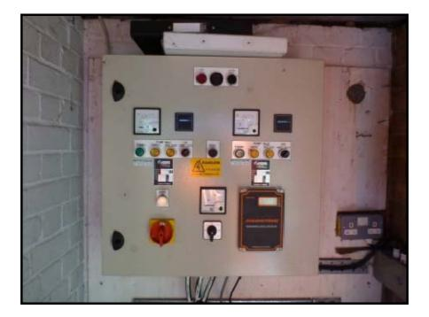
Figure 16 Pump Station Control Panel
