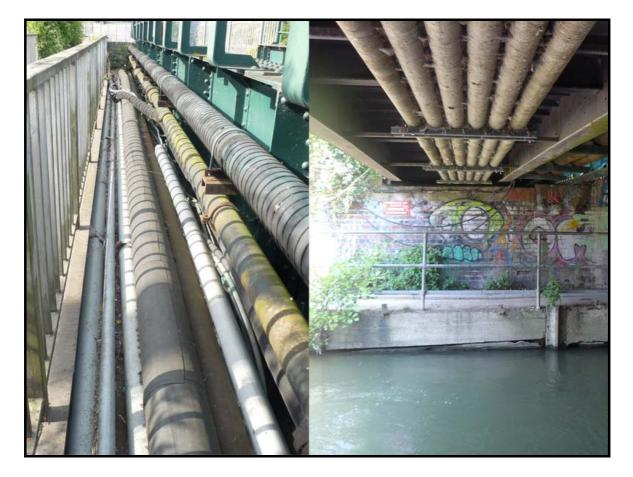
Figure 19 Sheepwash Bridge, Service corridor between deck 4 & deck 5 (left). Service ducts suspended below deck 5 (right)
