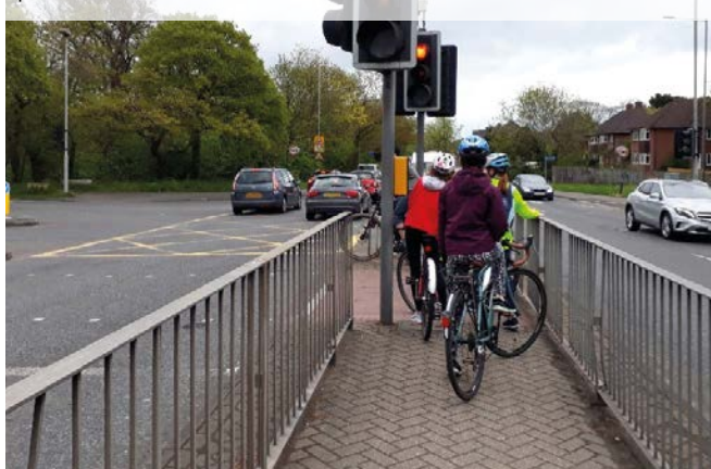
Figure 10.8: Toucan crossing with stagger – can be highly problematic
