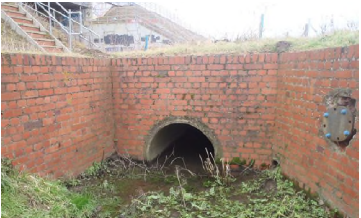
Figure 12 – Downside Elevation BGK/93 with Irrigation Main shown capped off
