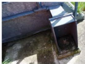
Foundation Connection - GV
