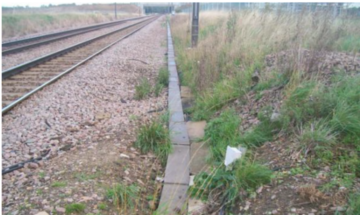
Figure 33 - Legacy route in poor condition and C/1/7 bypass route installed as part of FTN project.
