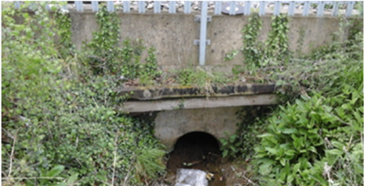
Figure 11 - Photo of Downside Headwall (SBR side)
