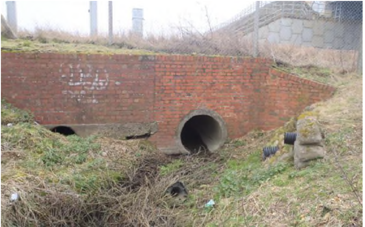
Figure 14 – Irrigation Main present in BGK/93 left culvert pipe
