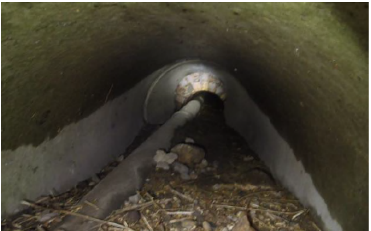
Figure 14 – Irrigation Main present in BGK/93 left culvert pipe
