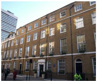
Figure 7.2 St. Thomas Street Facade - 1930's gap infilled between no. 8 and 10
