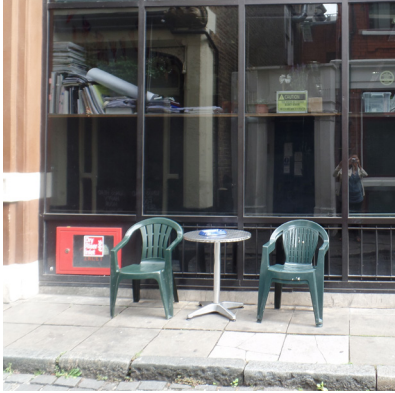
6. Low level obscure facade conceals the ground level floor zone & includes some service i.e. dry riser inlet.
