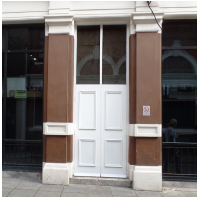
1. 1980s infill panels to resemble doors, fully sealed up - note insulation is visible to the rear of the smoked glass.
