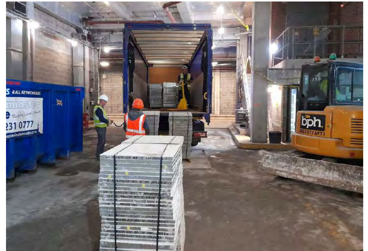
Fig: 15 Raised Access Flooring being loaded and sent to new building for refurbishment at a recent Cantillon project.
