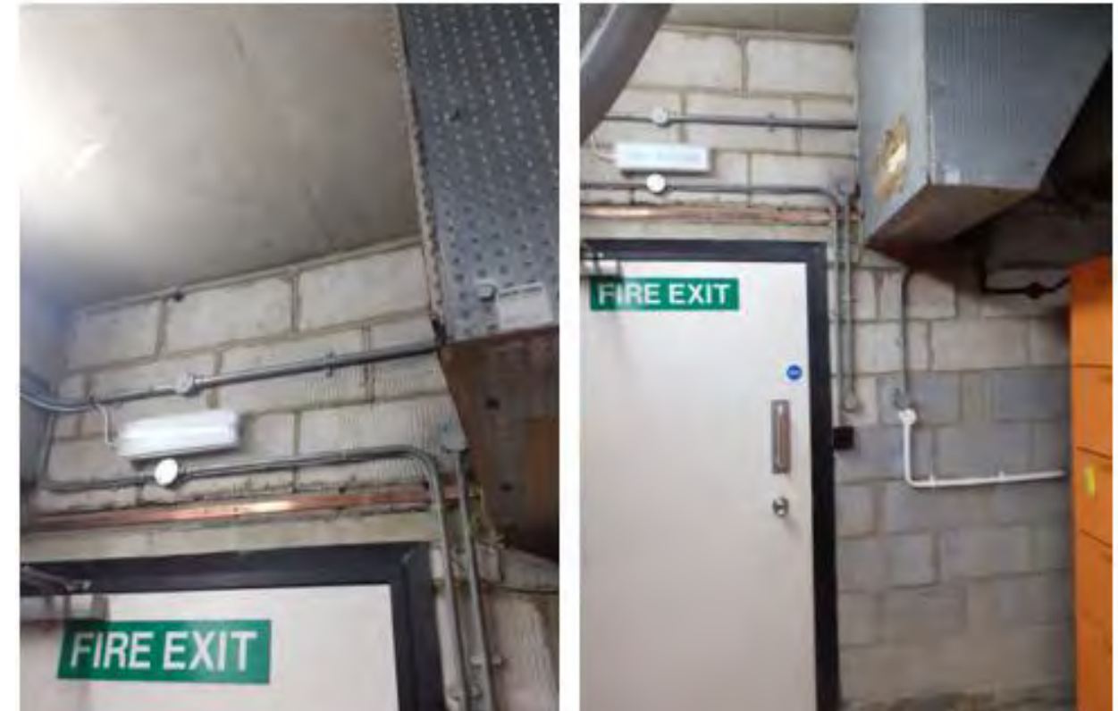
Fig. 1 Evidence of dense block wall construction within basement plant areas in New City Court
