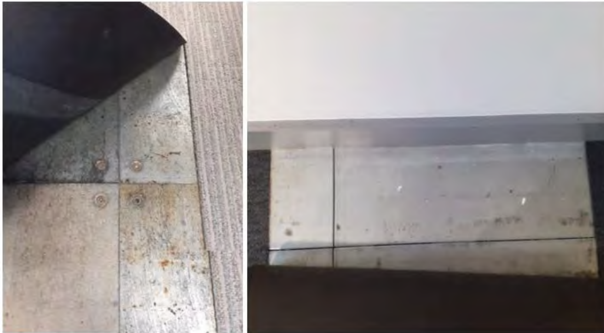
Fig. 2 Example of two types of Raised Access Flooring found in the building. (Left – Level 02 New City Court. Right – Georgian Terrace)
