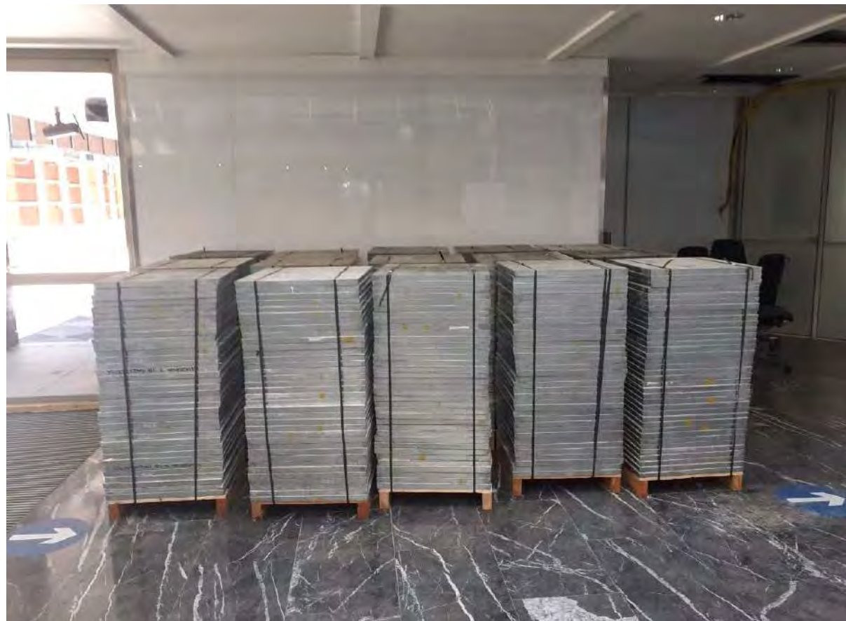
Fig: 14 Raised Access Flooring palletted at a recent Cantillon project.
