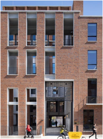
ESB Headquarters, Grafton Architects Note the set back brick facade at the final level, restrained use of materials and simplified Georgian proportions.
