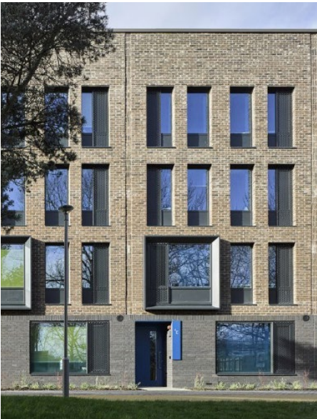
Cryfield Village, Warwick, RHP Note the variance in fenestration between floors, designed to identify the studio apartments as a different type to the smaller rooms on the floors above.
