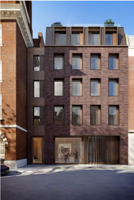
Gallery and apartment building, Studio Mackereth Note the interim metal panelled facade, providing a buffer for the overhanging cornice detail. Note the contemporary interpretation of a mansard roof detail, and the diminishing proportions of the windows.
