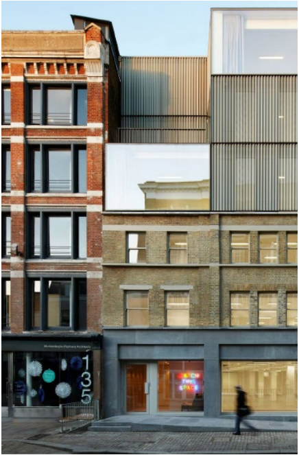
Curtain Road, Morris & Co A change of material to demarcate the final floors of the building
