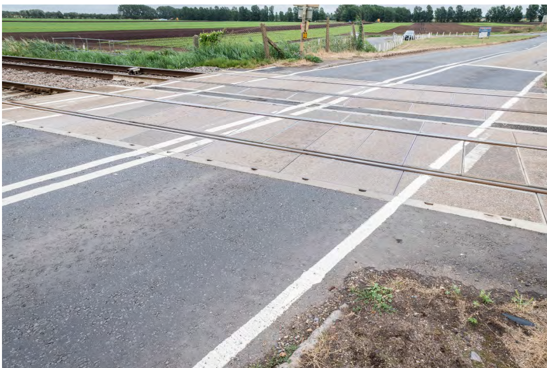
Figure 21 Crossing surface
