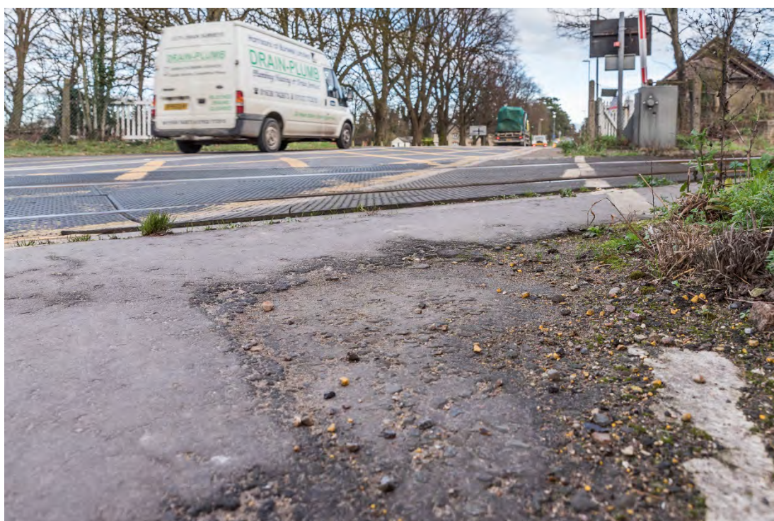
Figure 10 Footway trip hazard – South east side
