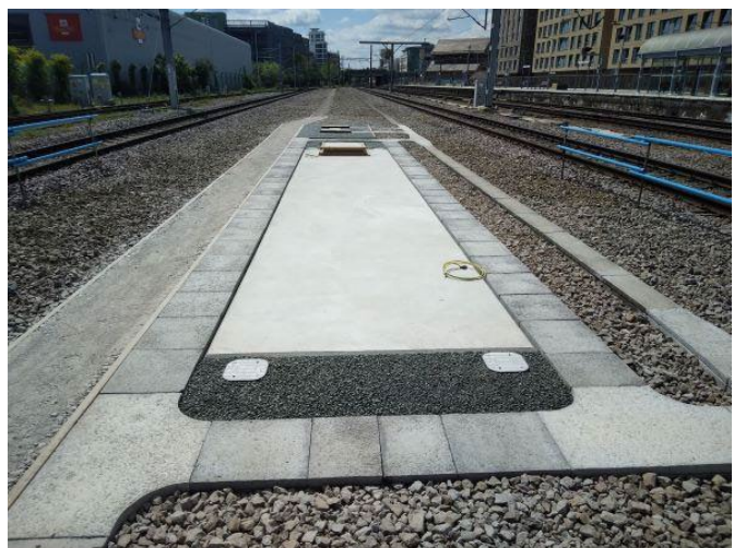
Figure 6 - Examples of SMIO Housing Bases plus surrounding landscape features and cable troughing
