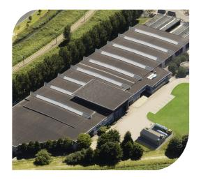
This is Indaver's cutting edge vegetable, garden and fruit (VGF) digester. It is the only machine in South Holland that can both digest and compost vegetable, garden and fruit waste, green waste and biowaste from the food industry and processes organic waste into green gas for around 3,000 households. Indaver recovers three valuable products from the process: compost, green gas and liquid CO2.
