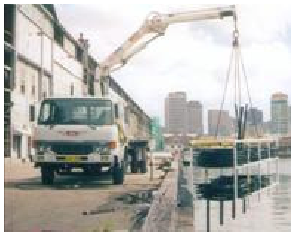
Figure 9: Laying 'flexible' pipework for a closed loop water source heat pump
