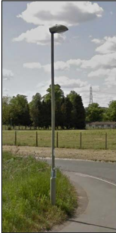
Figure 10 Post top mounted Urbis Sapphire lantern
