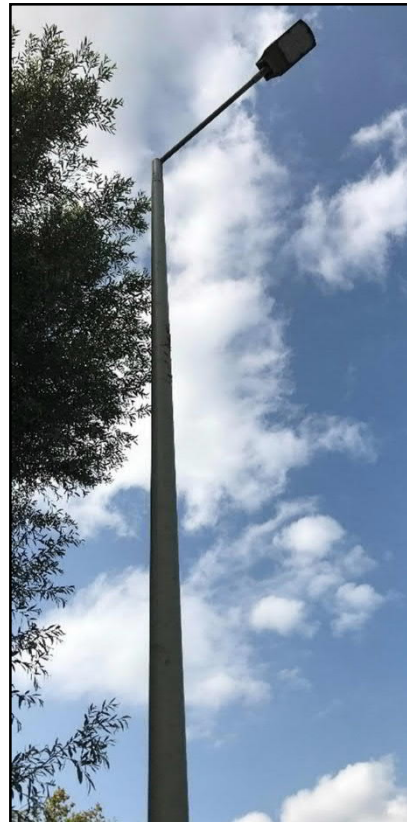
Figure 7 Side entry mounted SOX luminaire Figure 8 Side entry mounted LED ASD luminaire
