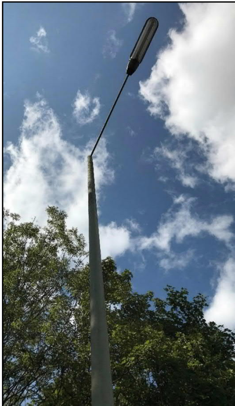
Figure 4 Side entry mounted SOX luminaire
