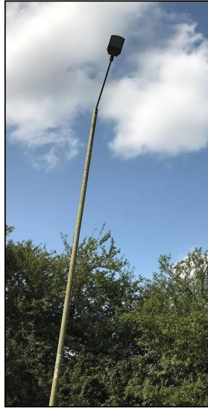
Figure 5 Side entry mounted LED ASD luminaire
