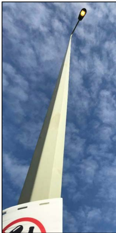
Figure 2 Side entry mounted Urbis Sapphire on 15m Octagonal tapered column
