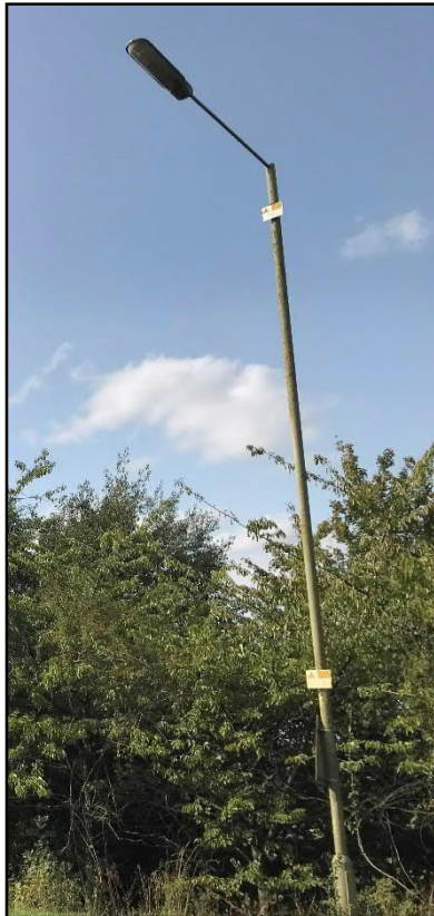
Figure 7 Side entry mounted SOX luminaire Figure 8 Side entry mounted LED ASD luminaire
