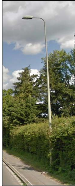
Figure 11 Side entry mounted Urbis Sapphire lantern
