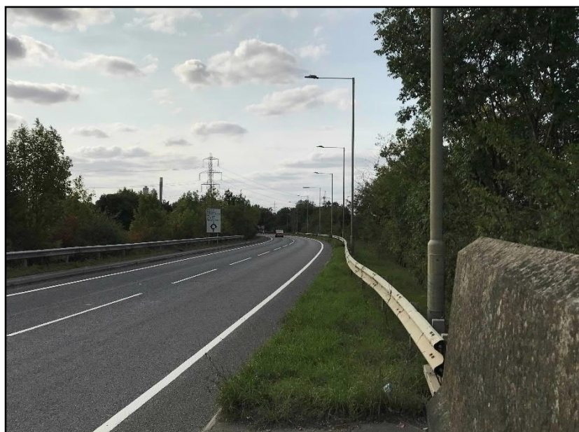
Figure 9 Street lighting arrangement behind VRS on the A4130 (East of Collett RBT)
