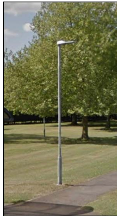
Figure 12 Post top mounted Urbis Axia LED lantern Figure 13 Post top mounted Urbis Axia LED lantern
