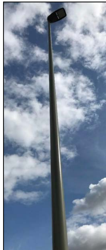
Figure 3 Post top mounted LED Kirium Pro luminaire on tubular steel column
