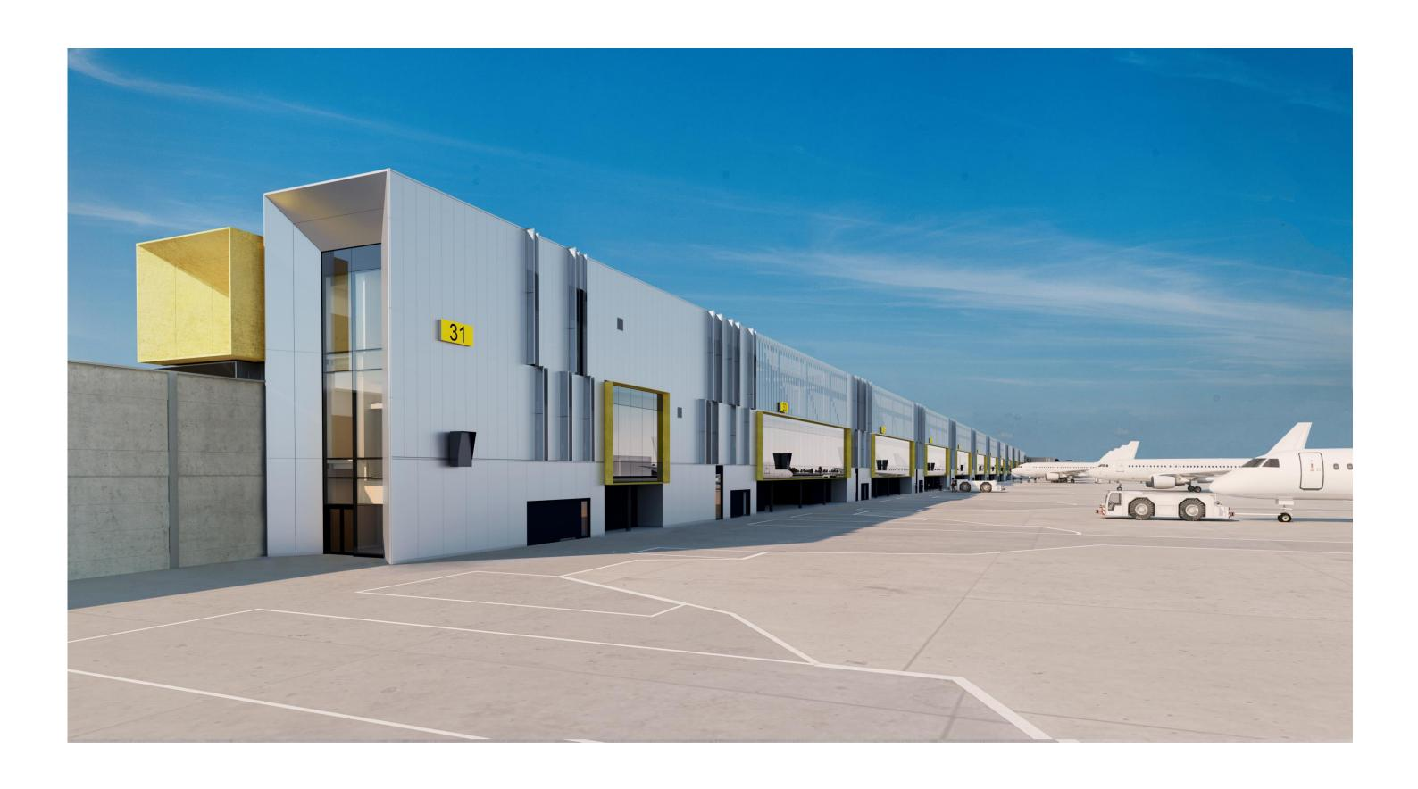
Figure 4.0.5: New Eastern Pier airside perspective view looking south-west - Proposed scheme without mesh to the solid areas of the façade and with exposed, enhanced composite panelling. Mesh is retained where the L20 roof plant areas, as per the approved scheme treatment.
