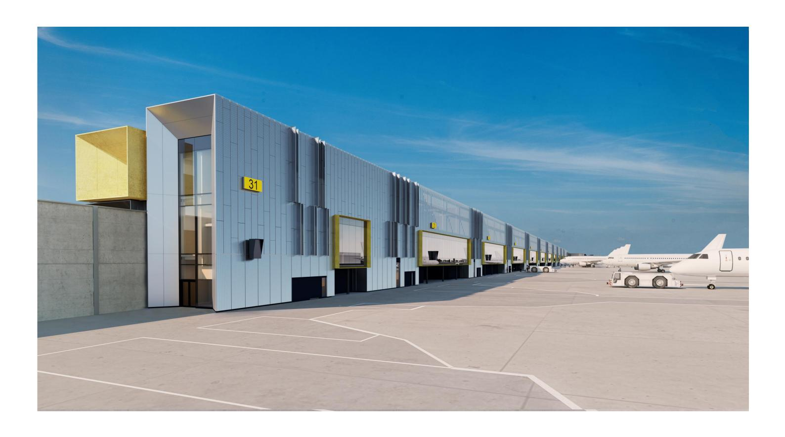
Figure 4.0.4: New Eastern Pier airside perspective view looking south-west - Approved scheme with expanded metal mesh over composite panelling.
