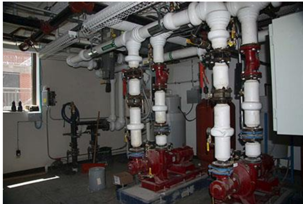
Ground source heat pump
