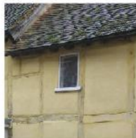
Light framing (studs) with render
