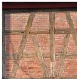
Light framing (studs) with brick
