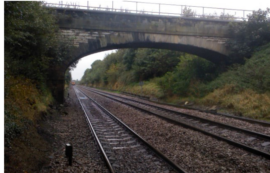
Figure 25: Brady Farm Bridge (HUL4/15). Design to span four tracks
