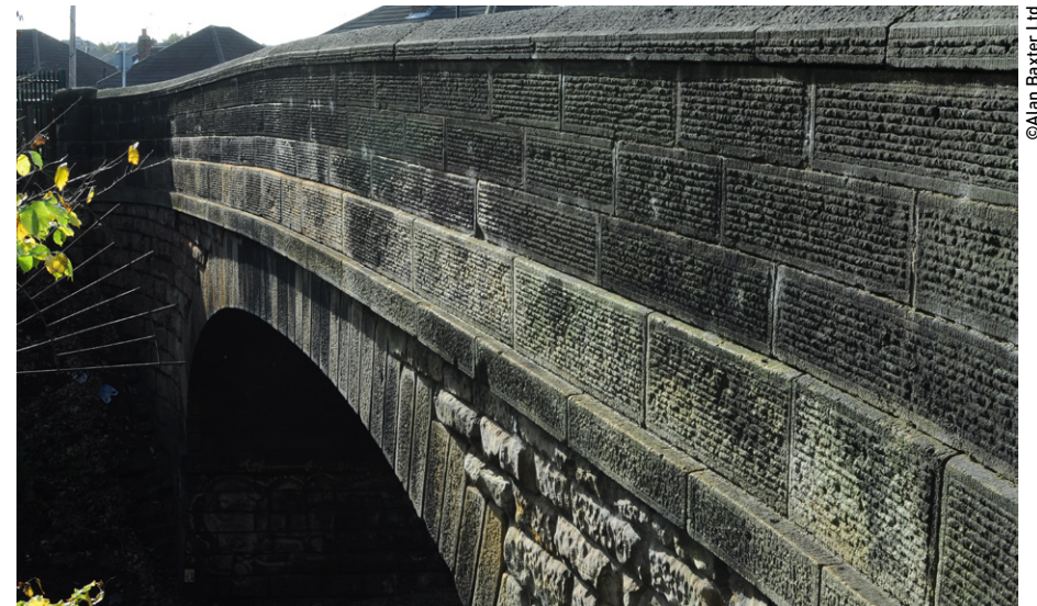
Figure 21: Example of the superb quality of masonry in Walker's bridge for the Leeds & Selby. This is Austhrope Lane (HUL4/21)
