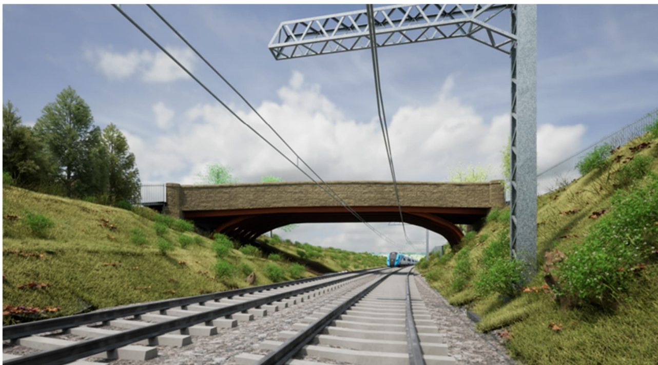
Figure 8 Weathered steel arch
