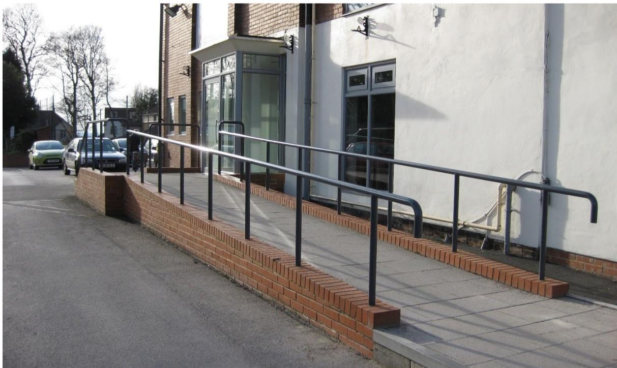
**Figure 38: Disabled Access Ramp Example**
