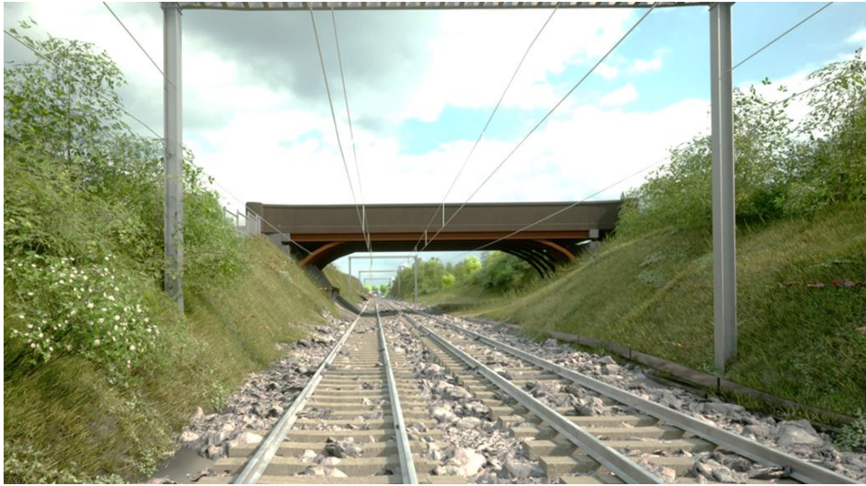
Plate 4 - Weathered steel arch
