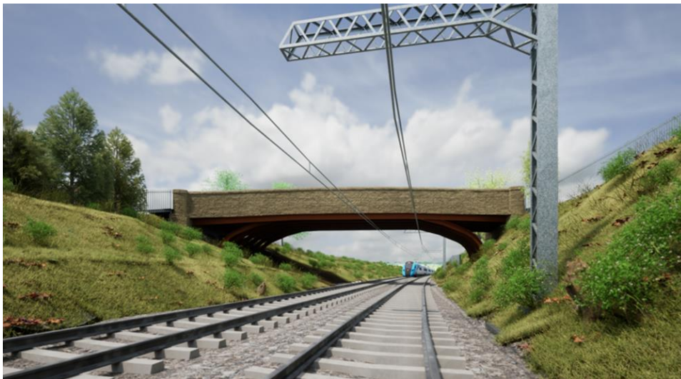
Plate 10 - Weathered steel arch
