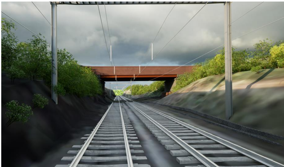
Plate 8 – Composite flat deck
