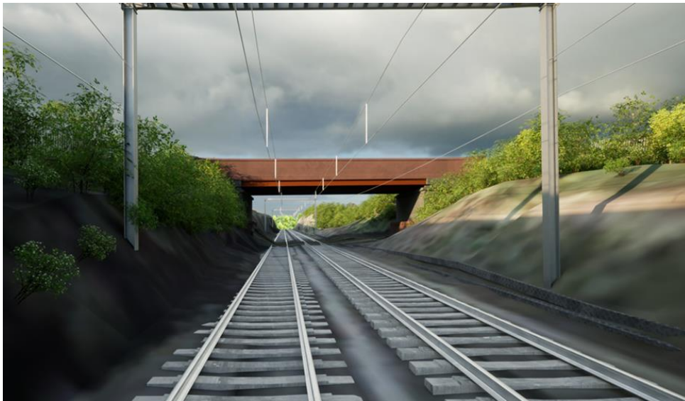
Plate 1 - Standard bridge reconstruction with stone cladding to parapets
