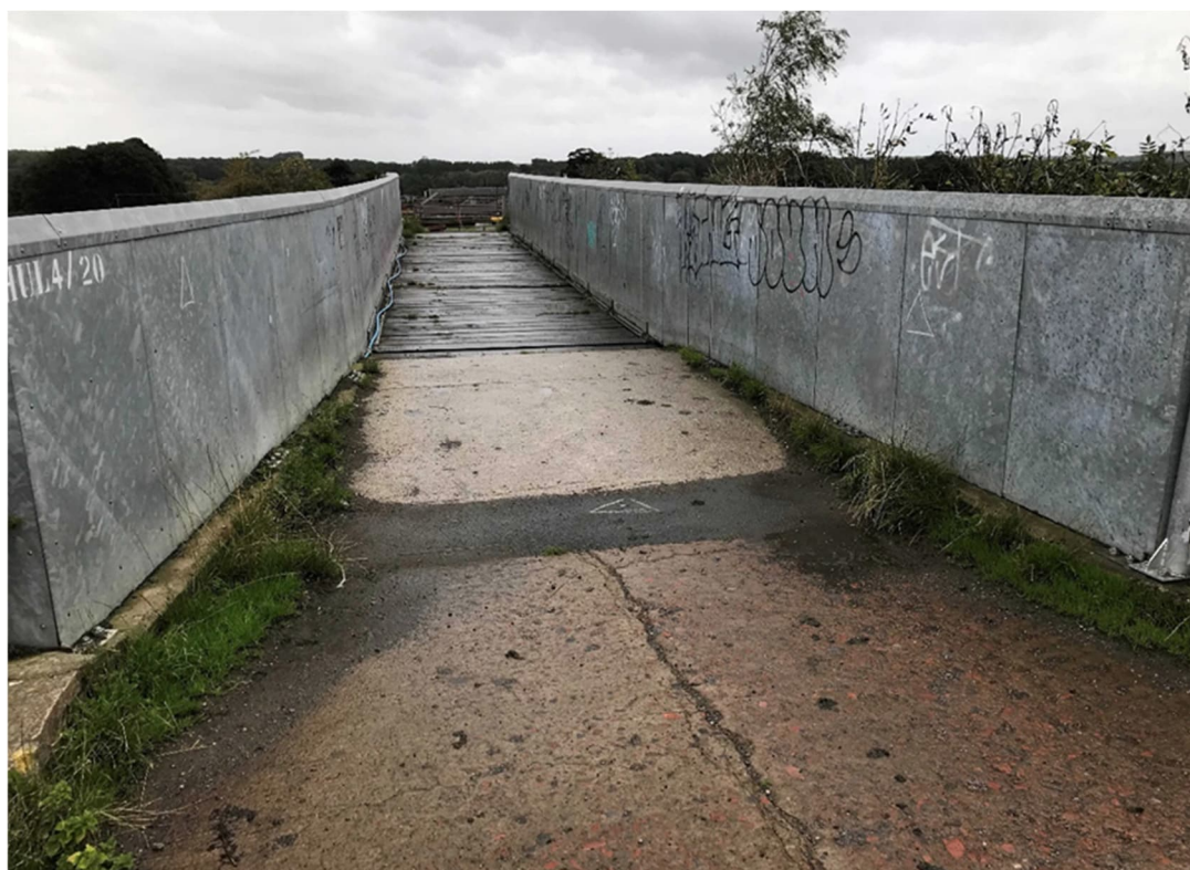
Figure 4 – Timber decking and steel parapets
